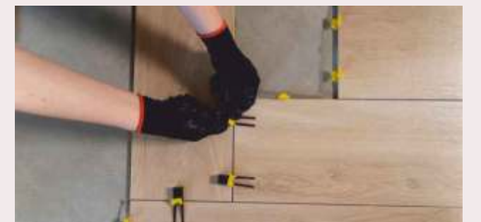
Extra care required in vertical pasting of Laminated sheet there is possibility of bubbles dueto lack of uniform pressure
